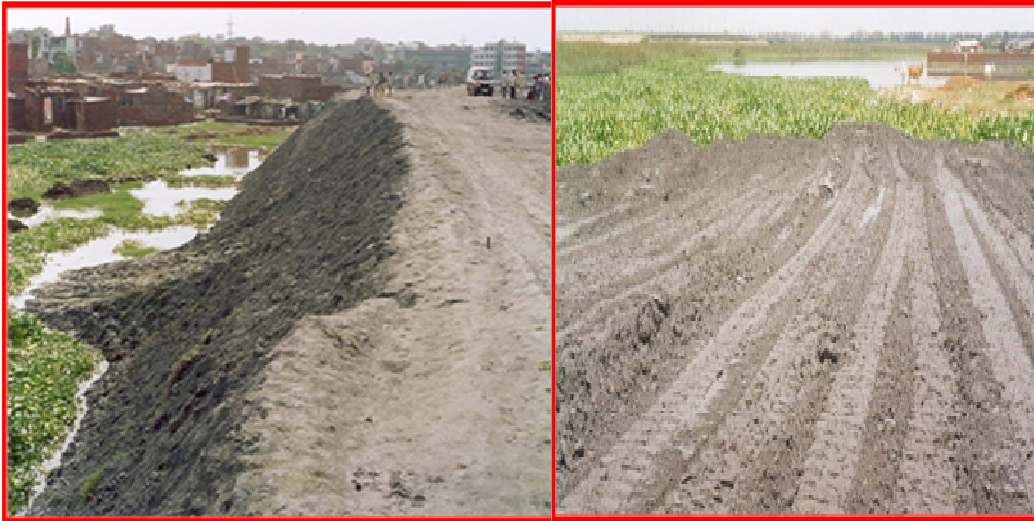
Fig. 1 Typical cross section of fly ash embankment construction is in progress
