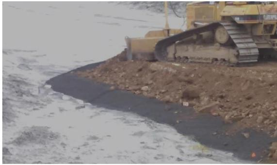
**Figure 13: Constructed drain with bottom ash and geogrid, Photo courtesy of R.B. Jergens**
