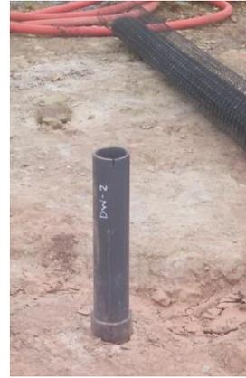
**Figure 12: Deep well at surface, prior to piping.**
