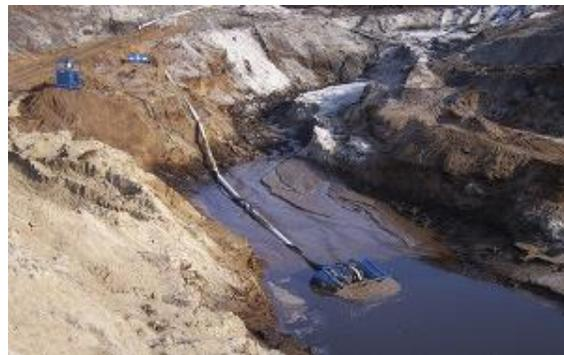
**Figure 10: Typical rim ditch with sump pump for drainage**
