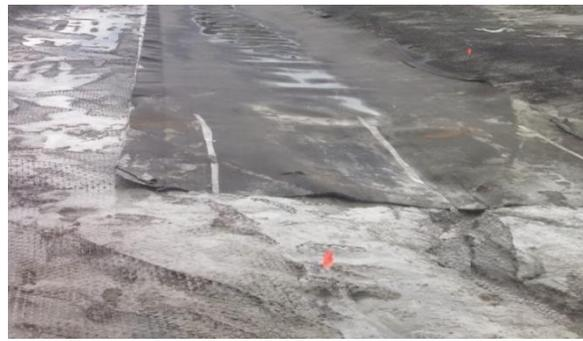
**Figure 14: Interior drain with geogrid, Coal Drain geonet, prior to bottom ash placement. Photo courtesy of R.B. Jergens.**
