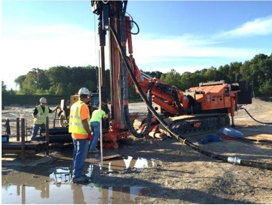
**Figure 11: Typical deep well installation. Photo courtesy of Moretrench.**
