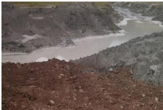
**Figure 9: Typical interior for rim ditch excavation**
