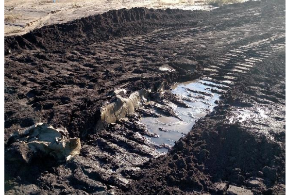
Figure 4: Track Hoe Bucket Penetration Test Located Near Porewater Transducer
