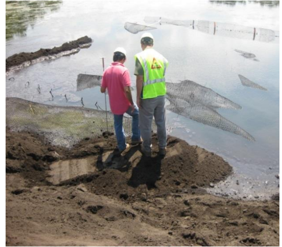
Figure :6 Hand held vane shear test readings safely obtained over geogrid
