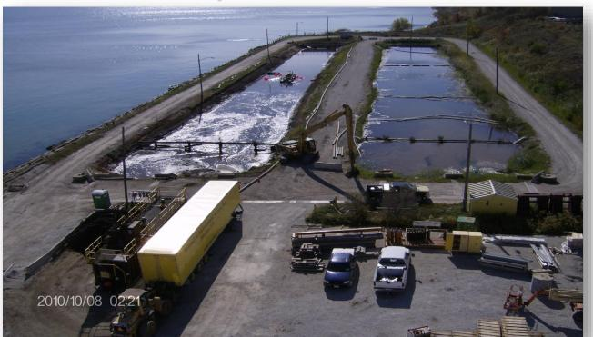
Question and Concern: Preliminary computations and current NPDES discharge requirements would require that the system would be 10 to 15 acres for a 45 acre site. How does the rate of treating dewatering water affect the rate at which ash can be excavated? Source: Project Photos from Metropolitan Environmental Services
